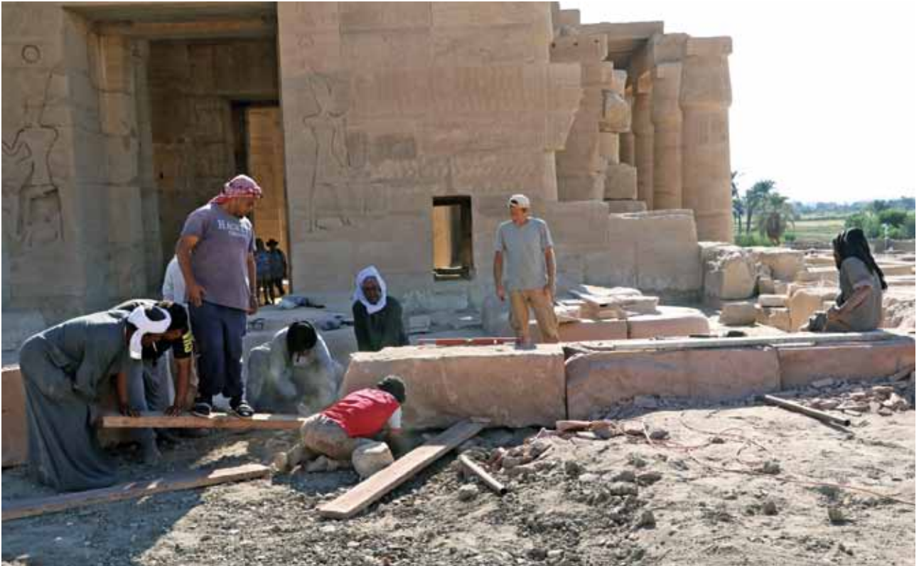
A.- RAMESSEUM. SECTOR ZSC (SANCTUARY). Restitution of the missing west wall of the Room of Litanies. (Photo © Ahmed Abdel Hamid Ahmed).
