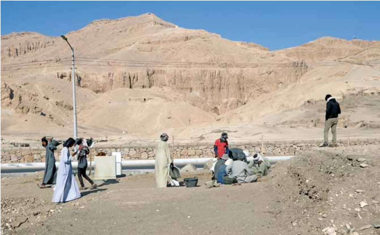
A.- RAMESSEUM. SECTOR APS. Cleaning the south-west corner of the External Enclosure. (Photo © Ahmed Abdel Hamid Ahmed).
